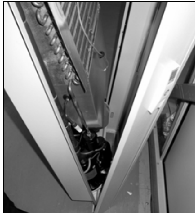
Fig. 8: Fit the climate control module in the section door
