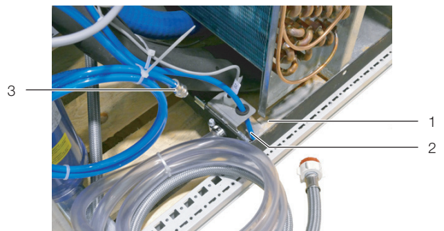
Fig. 63: Connections of the condensate pump
