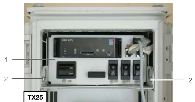
Fig. 22: Electronic module in the LCP
