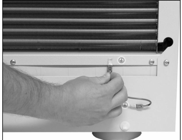
Fig. 25: Disconnect the earthing cable
