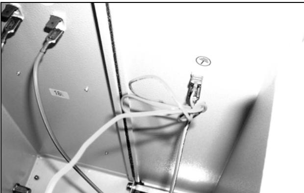
Fig. 68: Disconnect the fan earthing cable (1)
