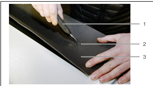
Fig. 6: Making the cable entry
