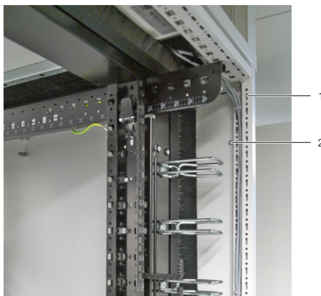
Fig. 10: Screwing the side panel
