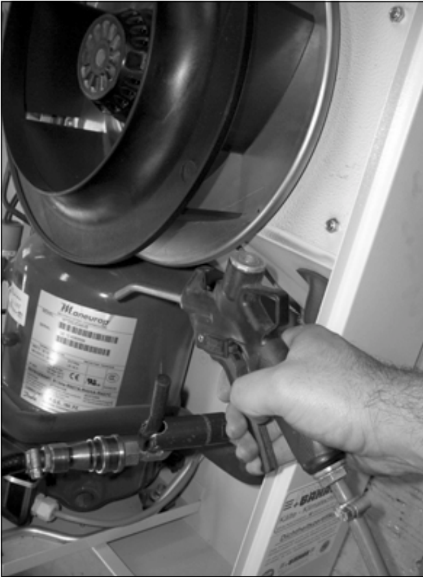
Fig. 59: Clean out the heat exchanger coil and compressor chamber using compressed air (2)
