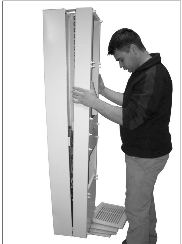
Fig. 78: Remove the cover
