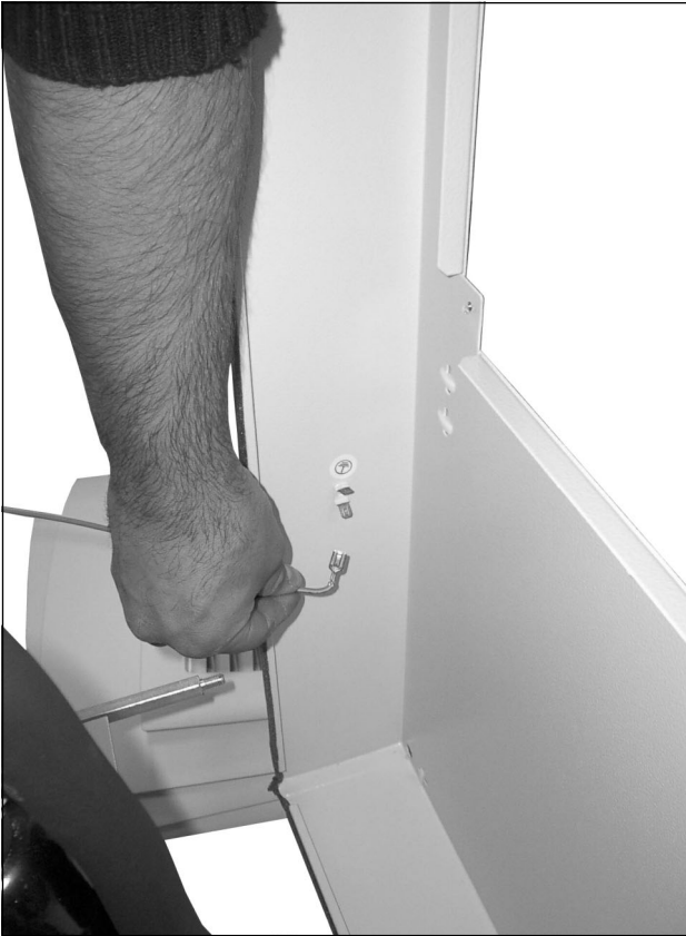
Fig. 80: Disconnect the earthing cable (2)
